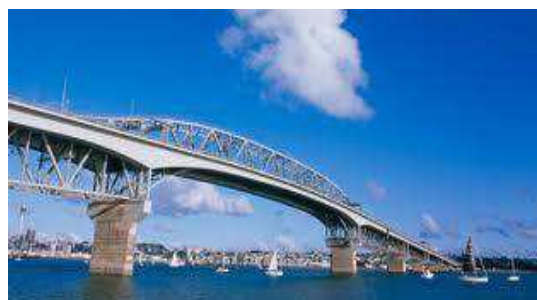
Auckland Harbour Bridge
